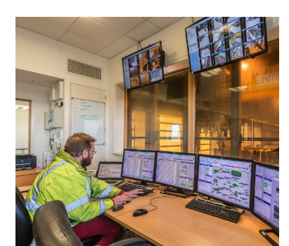
FLOW CONTROL SYSTEM
